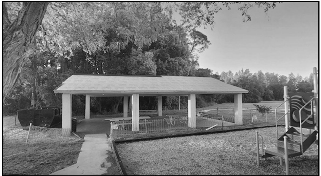
New roof going on park pavilion
